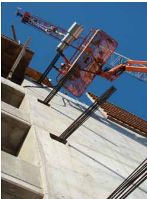
Collector beams on top of the shear walls were post-tensioned using between 19 and 38 strands per beam. This achieved a compressive force of 1.8 million pounds.
