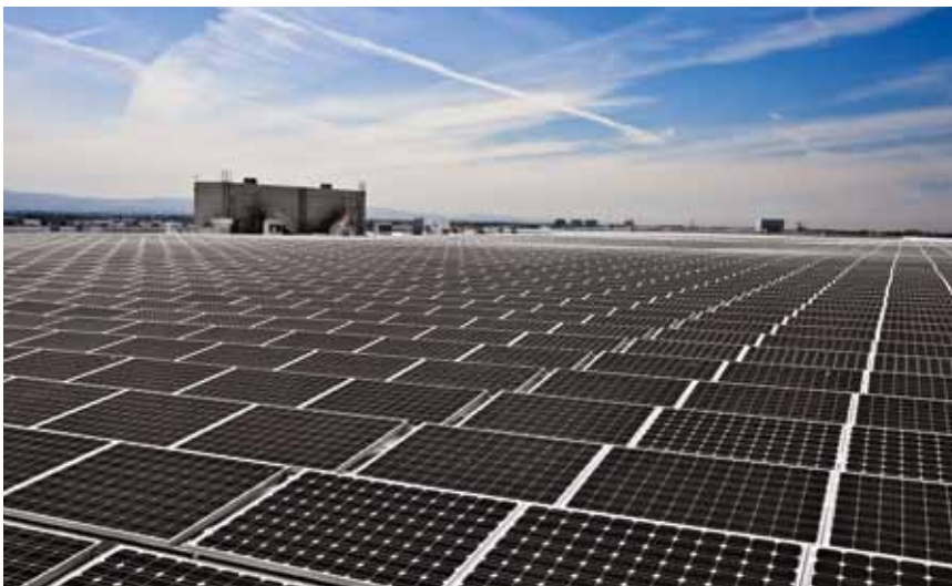
An array of 4,680 photovoltaic solar panels were installed on 3.4 acres of the roof to supply about 20% of the facility's electrical needs on an annual basis.
