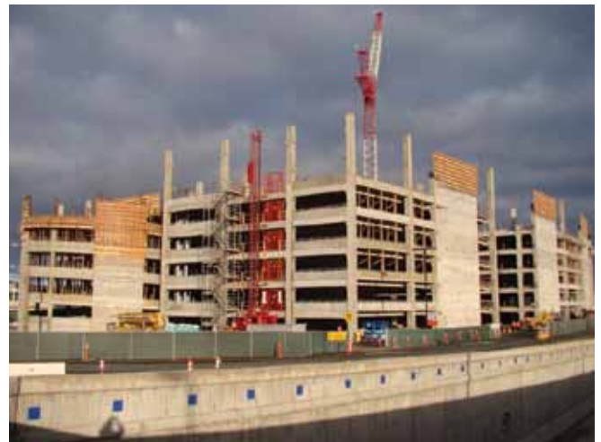
An M250 crane was used to erect the components, positioned at each corner as needed. The site was constrained both by airport activity and busy highways surrounding the airport.
